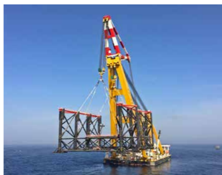
4 FLOATING SHEERLEGS AND CRANE BARGES
