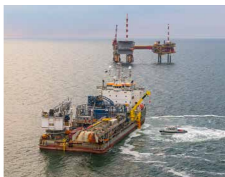
4 CABLE-LAYING VESSELS AND BARGES
