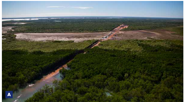
A Shore approach during construction B SSDV Ndeavor
