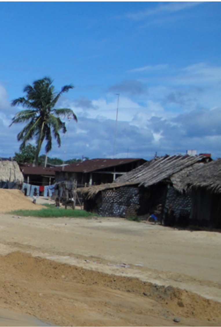
FORCADOS / OGULAGHA Coastal defense project during which a total of 2,300 meters of coastline was raised and reinforced in order to protect the fishing village of Ogulagha near Forcados
