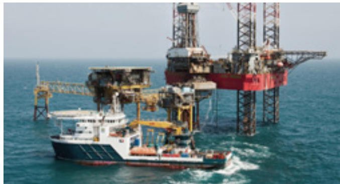
from top to bottom: Diving works
