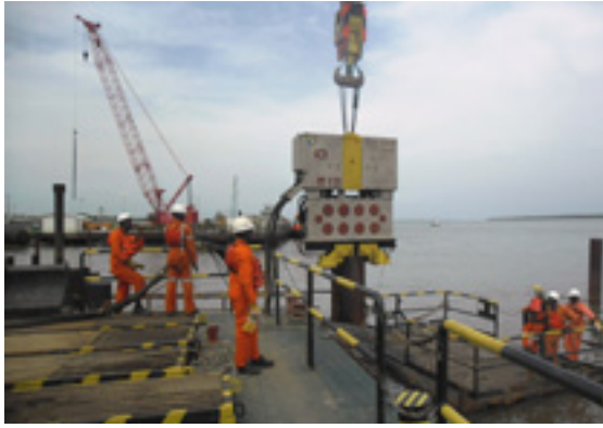
ESCRAVOS Driving sheet piles for the cofferdam at the EGP3A landfall site at Escravos
