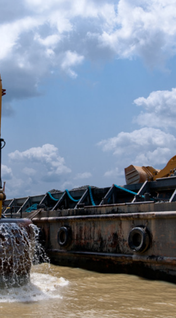
Backhoe dredger Ilajeland
