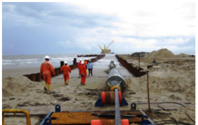
ESCRAVOS Pipe pull for Chevron Nigeria's EGP3A project
