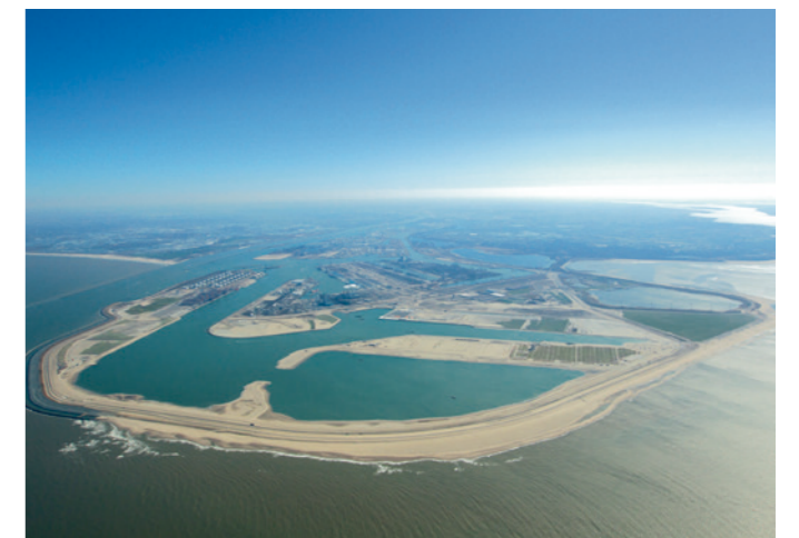
ROTTERDAM, THE NETHERLANDS Maasvlakte 2 Port Expansion. Innovative Design, Construction, Maintenance. 700 hectares, 11km of sea defense, 3.5km of quay walls, 14km of roads and railways. Numerous interfaces, strict design, environmental and safety challenges were successfully met.
