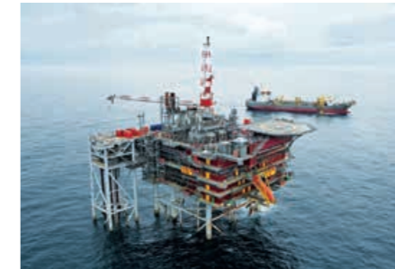
DE RUYTER FIELD, THE NETHERLANDS Seabed preparation works, with the Trailing Suction Hopper Dredger the Oranje, for pipeline installation and burial.
