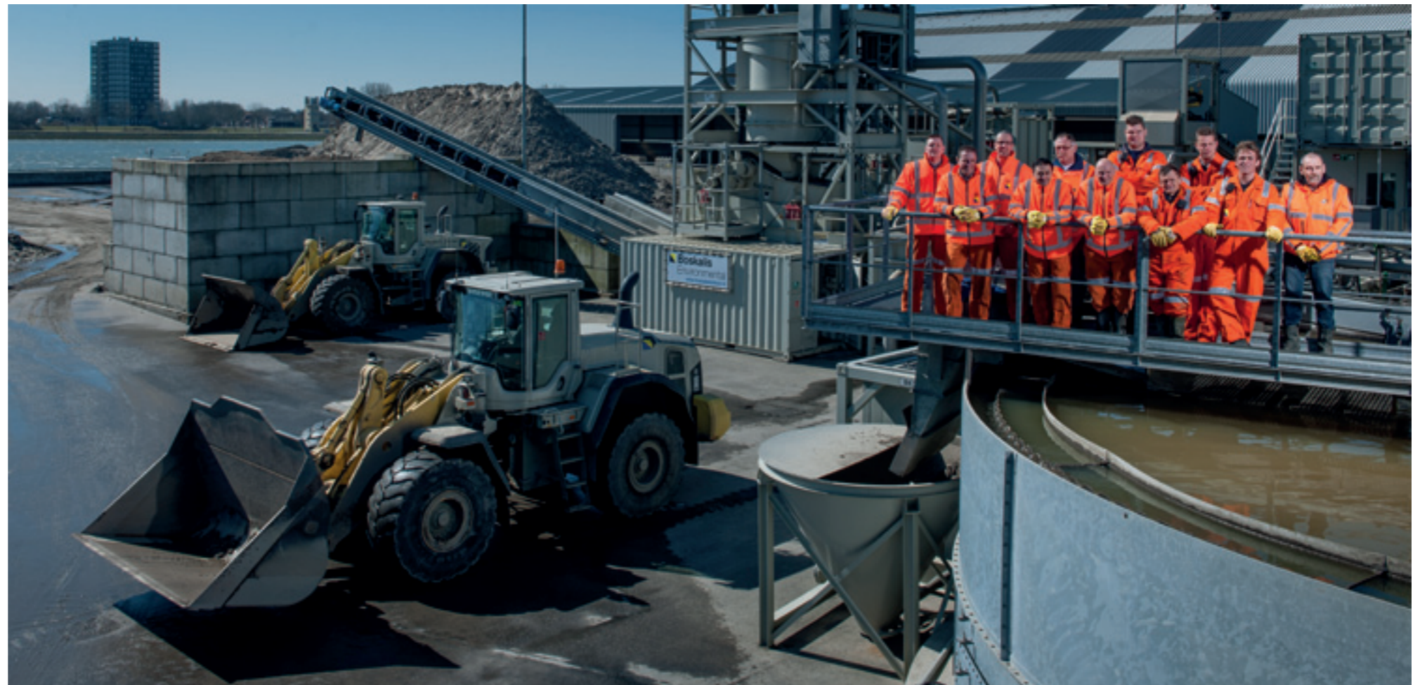
SCHIEDAM, THE NETHERLANDS Operational team at the permanent soil treatment site.
