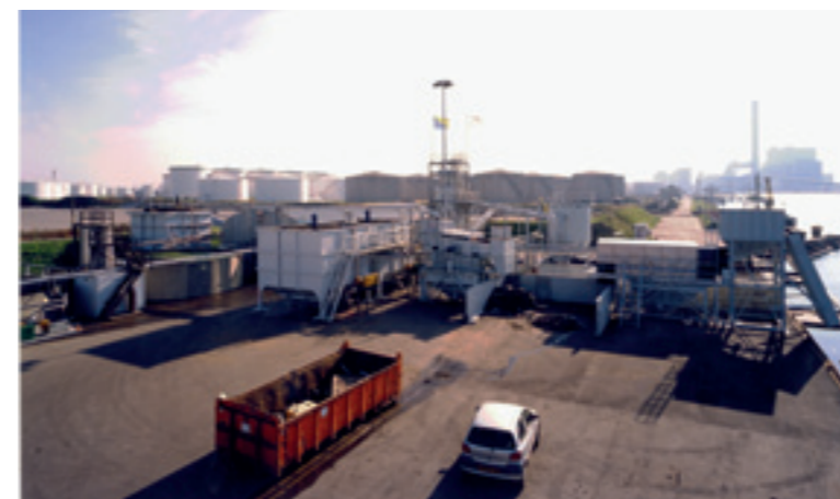
bottom left ROTTERDAM, THE NETHERLANDS Aerial view of the 'Slufter' Confined Disposal Facility. The 'Slufter' is a large scale CDF for the disposal of contaminated sediments.
