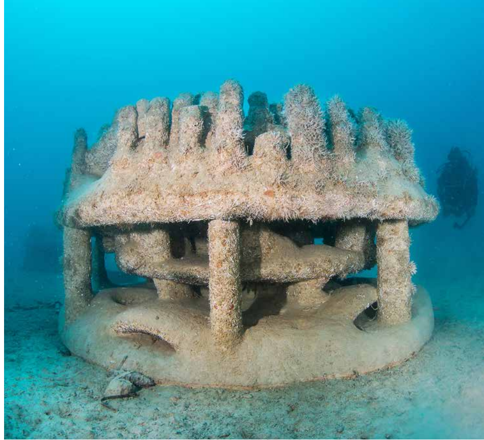
ARTIFICIAL 3D REEFS PRINTED FROM LOCALLY DREDGED SAND AND DESIGNED SPECIFICALLY FOR THEIR ENVIRONMENT, CREATING AN OPTIMAL HABITAT FOR LOCAL CORAL DEVELOPMENT.
