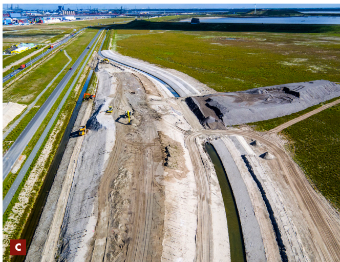
C Application Amaliaviaduct Maasvlakte
