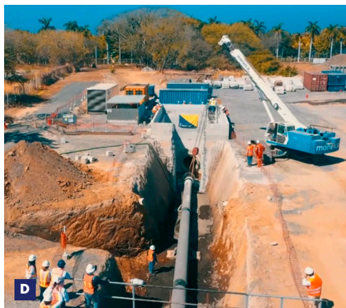
D Pipe pull through micro-tunnel E Diving activities F Berthing of a LNG tanker
