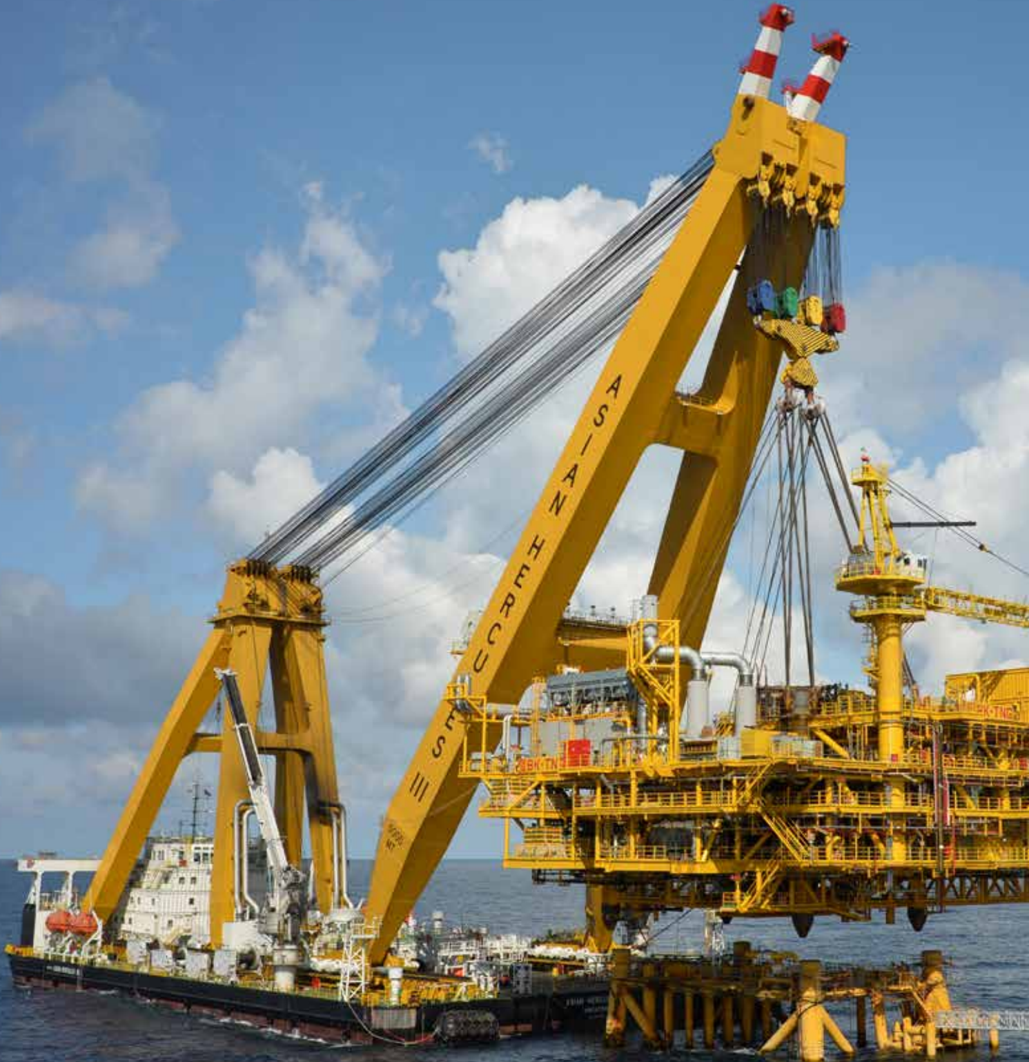
Installation of the 4,200 ton Thien Ung platform topside by the sheerleg crane Asian Hercules III offshore Vietnam.
