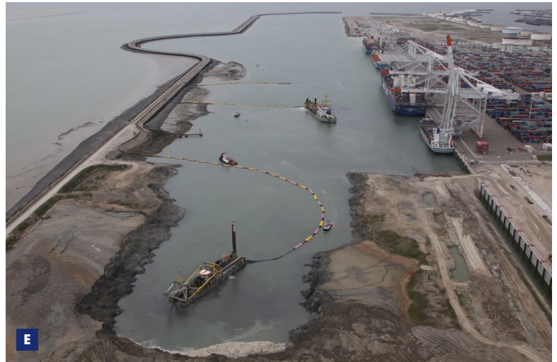
C Dredging close to the quay wall
