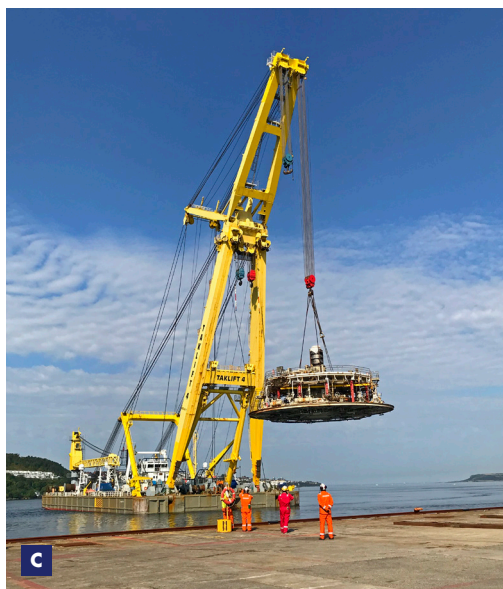
C Lifting of turntable
